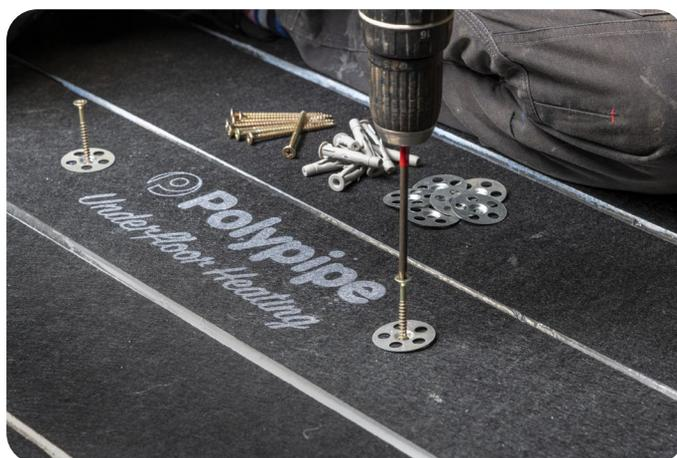
Depending on the type of substrate, the Polypipe Overlay™ Plus or Polypipe Overlay™ Plus Acoustic can be fixed with screws and washers or a continuous bed of flexible tile adhesive. It is essential that the floor onto which the panels will be fixed are flat and exhibit no movement. An uneven floor must first be made flat using a levelling compound.
